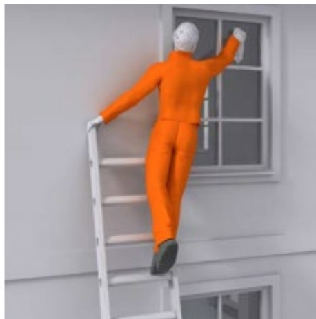
Incorrect use – excessive stretch and missing 3 contact points
