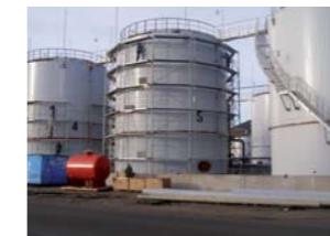
VKG Oil AS renoveeritud mahutitepark.
